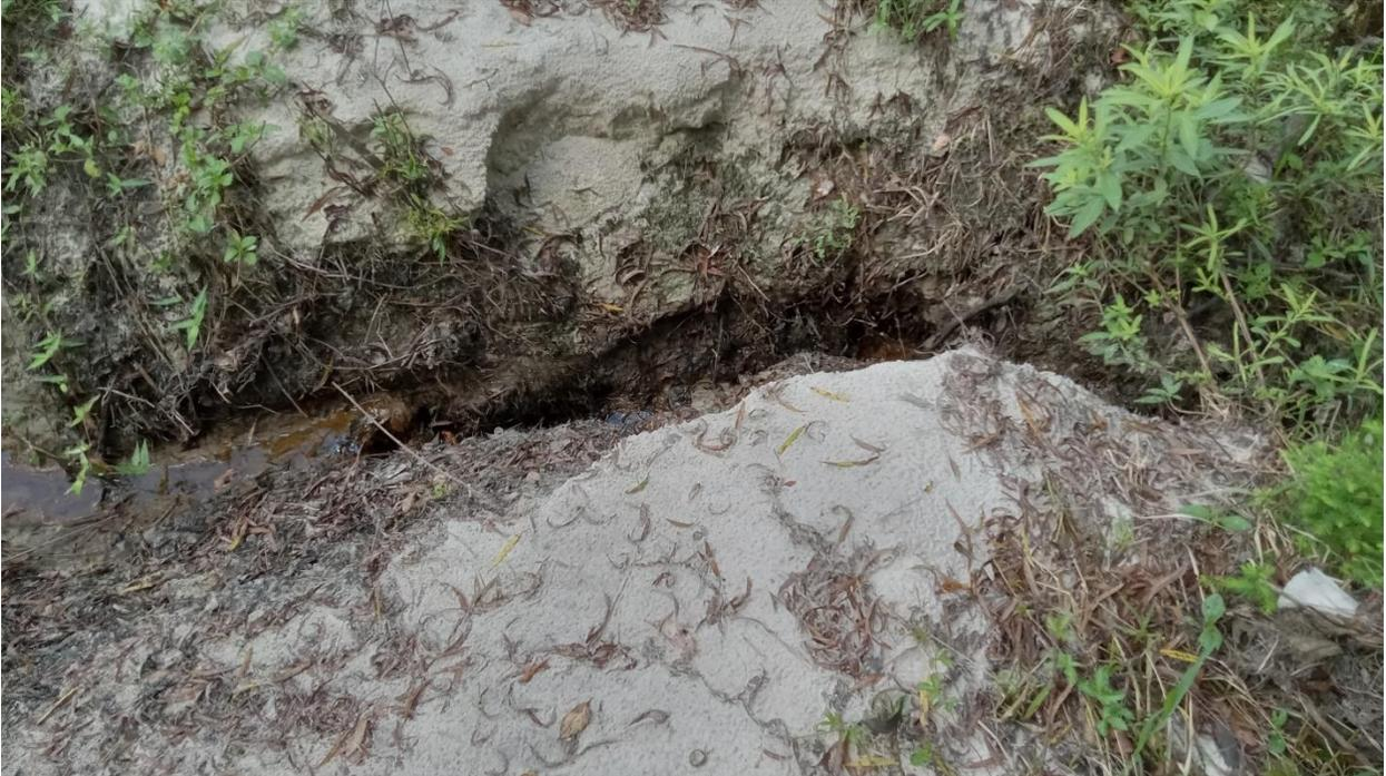
Small eroded area that lets water pass into and out of the constructed wetland. Image is from 8/30/2024/
