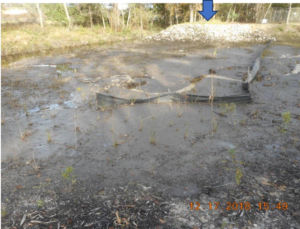
Blue arrow shows where the old service road that went along Alligator Creek to the pipeline utility crossing was located. The road was removed to create the wetland area.
